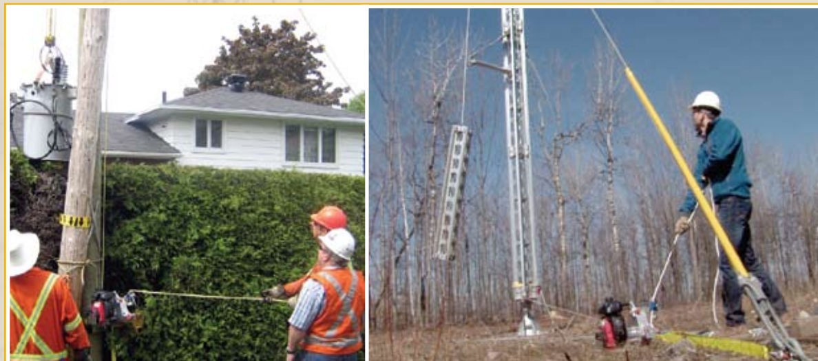
LIFTING EQUIPMENT, TRANSFORMERS
