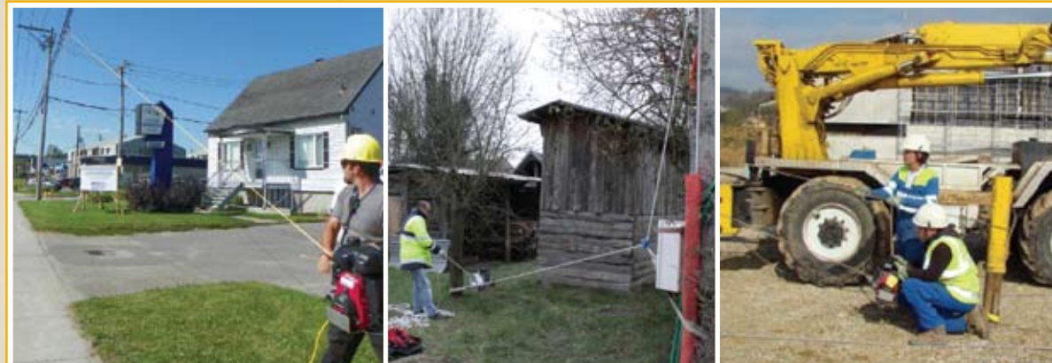
PULLING WIRES, FIBER OPTIC OR CABLES
